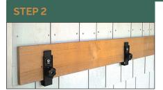
Choose a straight ledger board, 3/4 inches thick, previously cut to the width of your exposure. Insert it into the installation tools, taking care not to dislodge them (see Figure 2).
