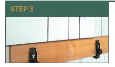
Install the cedar shingles by placing them on top of the ledger board while following the SBC cedar shingle installation instructions. Once the shingles have been nailed or stapled, remove the board and the tools, then return to step 1 (see Figure 3).
