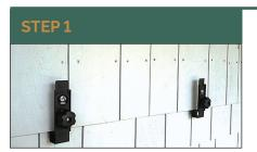
Slide the Easy Installation Tools retention legs up and behind previous course (see Figure 1). Make sure the tool stop is tight against the butt edge of the shingle. To do so, simply tap under the tool with a hammer.
